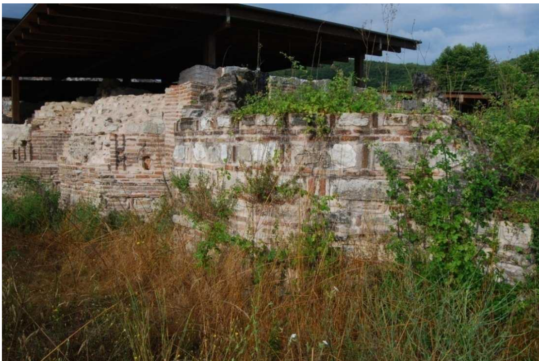
Figure 41 : Pantanassa Philippiados, eastern facade (Georgiadou, 2015 : 457).
