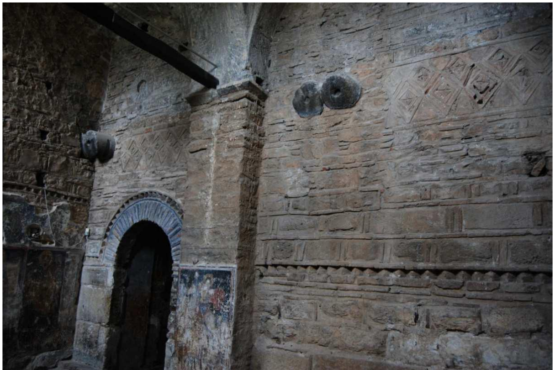
Figure 66 : Paregoretissa, Arta: Detail of the exterior north wall of the main church (photo: R. Ousterhout). (Georgiadou 2015, 478).
