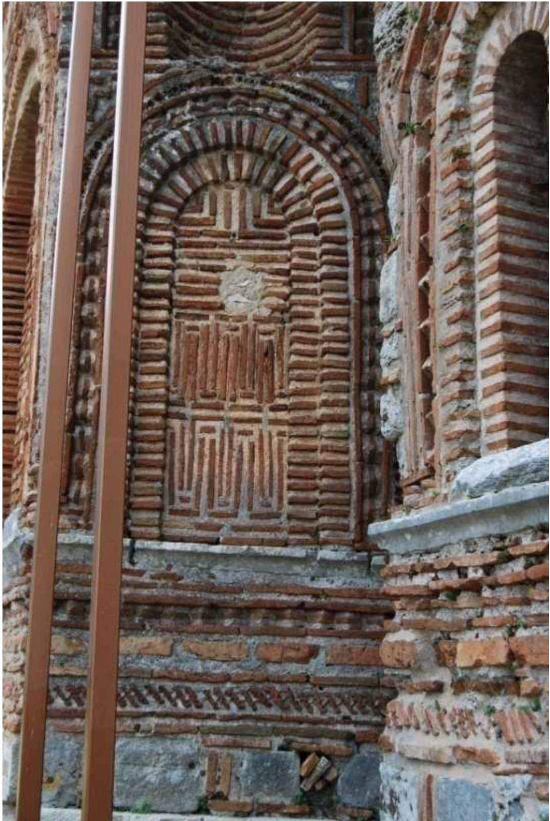
Figure 62 : Paregoretissa, Arta: Detail of the north side of the central apse (photo: R. Ousterhout) (Georgiadou 2015, 475).
