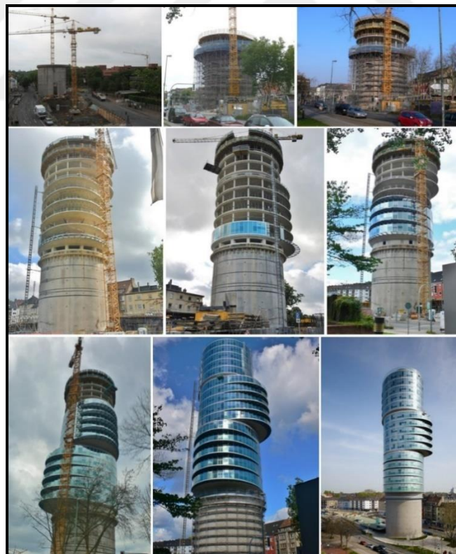
Figure 5.51. Construction stages of transformation of Rundbunker to Exzenterhaus 2008-2013 [182].
