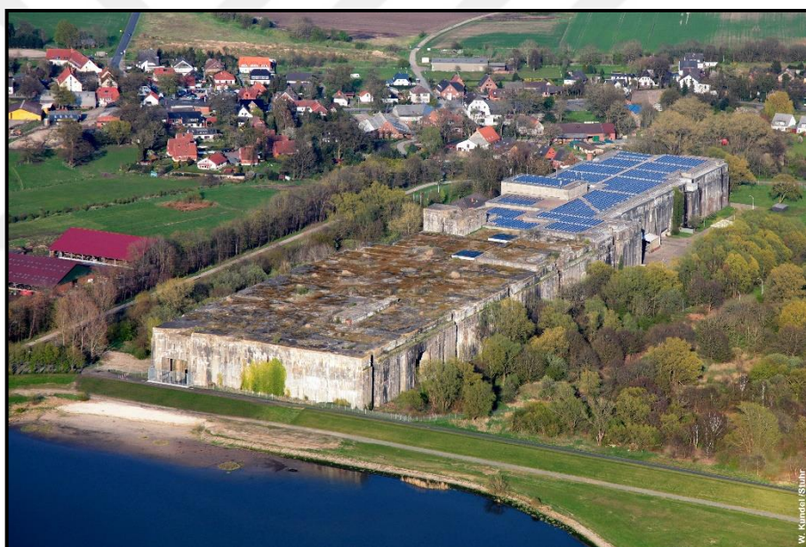
Figure 3.29. Valentin Hochbunker 8 submarine and ship factory 1943-1945 present state, Bremen [80].
