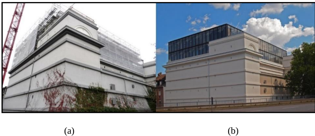
Figure 5.58. (a) Photo of construction of Hochbunker at transformation, (b) photo of after add two floors in the Hochbunker [191], [192].
