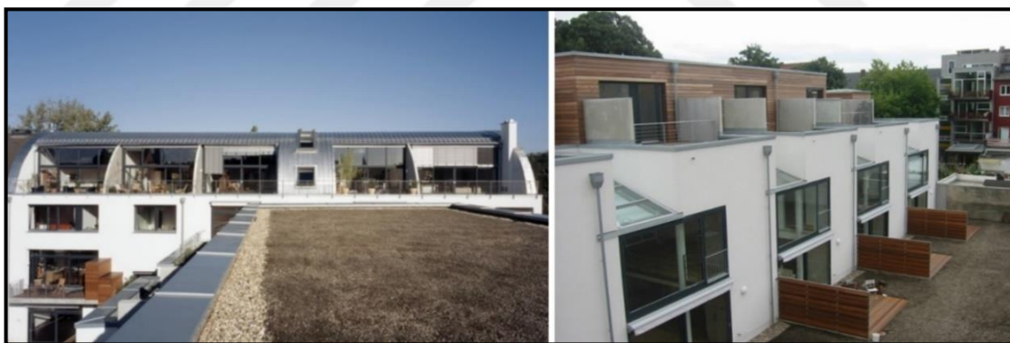
Figure 5.11. Rooftop after transformation at Hochbunker, photo by Constantin Meyer [137].
