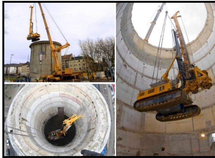
Figure 5.50. Insertion of drill rig into Hochbunker with telescopic crane for pile foundation placement [177].
