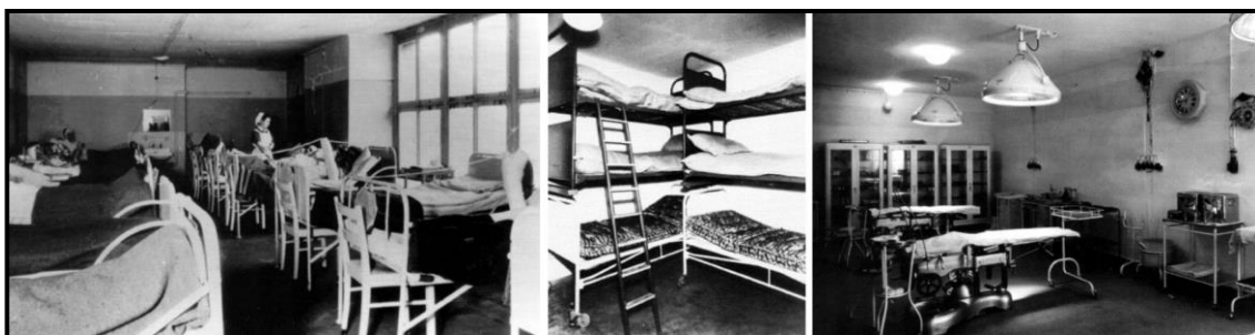
Figure 3.34. Hospital Hochbunker interior photos, the initial photo is general hospital layout, the bunk bed layout in the middle, the photo of the order passed as a result of the increase in the number of injured and patients coming to the hospital, Operation room photo [20].
