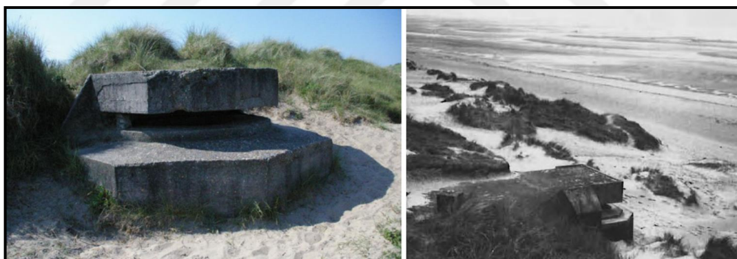
Figure 3.40. Photo of Telephone Bunker [39], [85].
