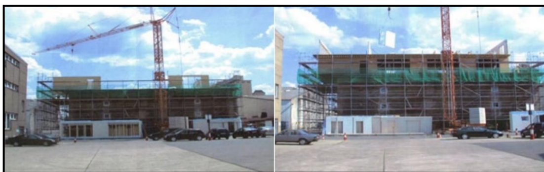
Figure 5.24. Photo of construction of two new floors [141].
