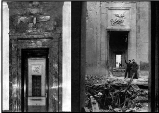
Figure 2.16. Nazi building in Germany before photo and after photo of the end of the war in 1945 [32].
