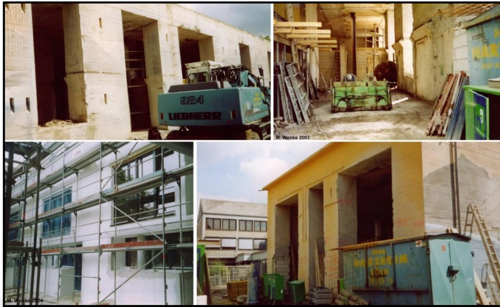
Figure 5.16. Construction of Hochbunker between 2002-2003, photo by M. Wenke [135].
