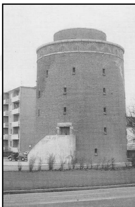
Figure 3.14. Example of openings at Hochbunker; entrance and small window openings [72].
