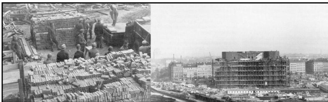
Figure 5.62. Construction of Feldstraße Bunker 1942 [36].
