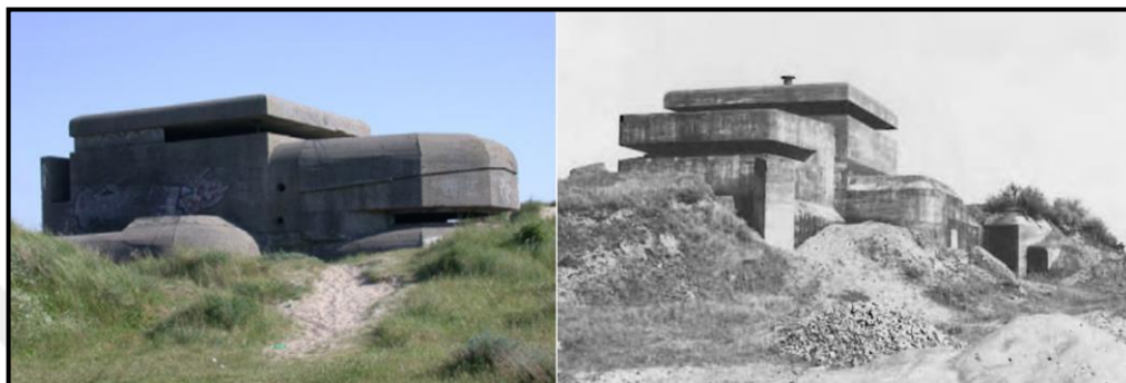
Figure 3.37. Photos of Fire Control Bunker [39], [85].
