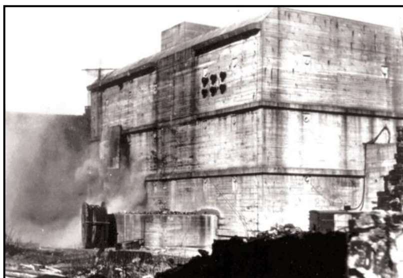
Figure 4.5. Hochbunker demolition, Emden [88].
