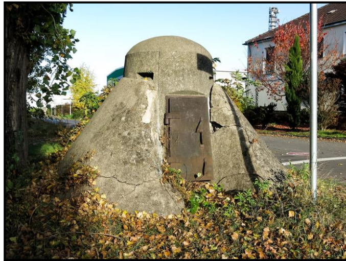
Figure 3.11. Small size bunker, "Einmannbunker" Bonn in Maarstrasse [65].
