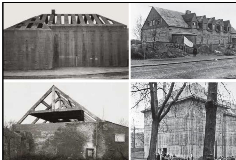
Figure 3.17. Camouflage Hochbunkers example, similar roofs of the surrounding buildings. (1942-45) [24], [74].
