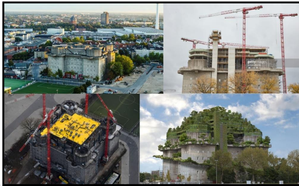
Figure 5.66. Hochbunker construction photo by Georg Wendt [199], [200], [201].
