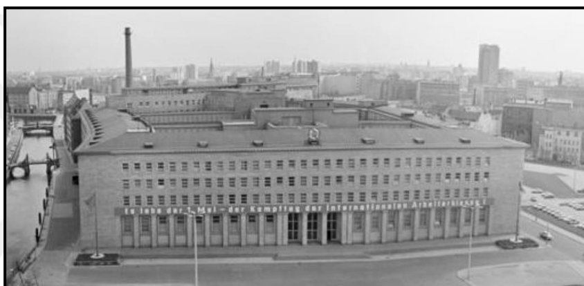
Figure 4.6. The Ministry of Finance Building in East Berlin [89].
