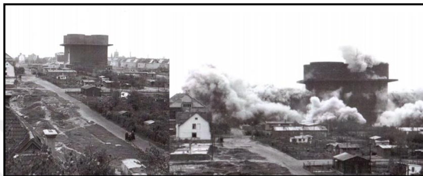
Figure 5.35. Gefechtsturm VI, Wilhelmsburg, inner walls destroyed on 17 October 1947 by the British army's [34].
