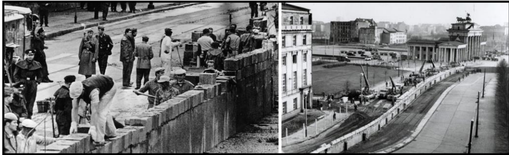
Figure 2.22. Berlin Wall construction 1961 [54], [55].
