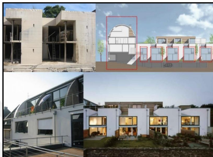
Figure 5.12. The left photo at the top shows the openings at construction. The right photo of the top is a cross-section. Photo of under side show the after look to transformation at the Hochbunker, by Thomas Luczak and Constantin Meyer [137].
