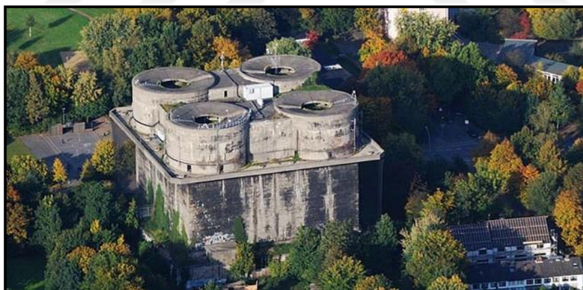
Figure 5.36. The Hochbunker before look of transformation to Energy Bunker, greening facade of Flak Tower [169].
