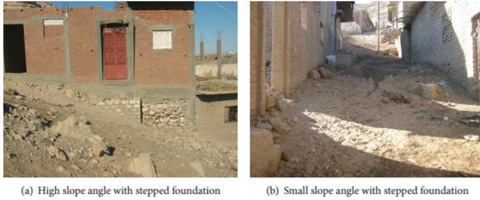
Figure 4.42 : The techniques of constructing building on hillside slope in Doronka village (Farghaly, 2014).
