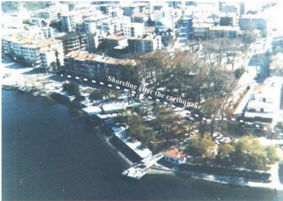
Figure 5.56 : View of Degirmendere nose before the earthquake (Cetin et al,2003).
