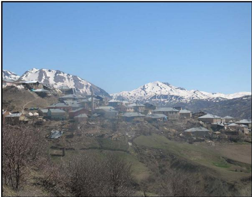
Figure 3.6 : A general view of damaged Okçular village (Yilmaz & Uran, 2010).
