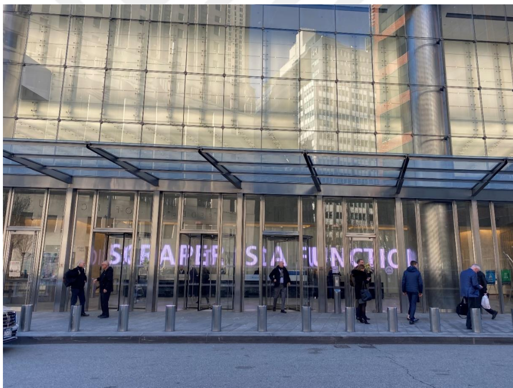
Figure 13: Current date of pictures, February 11, 2020
