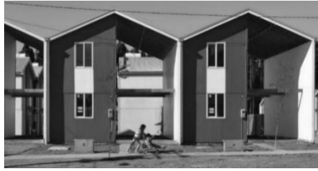
Figure 4.5. Voids that are not juxtaposed in Villa Verde Housing units (Elemental, 2013)
