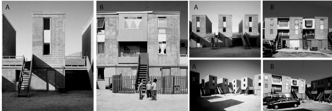
Figure 3.24. Quinta Monroy Housing Project before customization and post-customization of users ("Quinta Monroy / ELEMENTAL", 2008)
