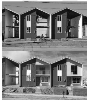
Figure 4.2. “Half of a good house” (top) and “Middle-class standard achieved by the residents themselves” (bottom) (“The Pritzker Architecture Prize 2016 Laureate Alejandro Aravena”, 2016, p. 28).
