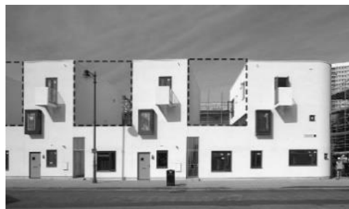
Figure 2.4. Donnybrook Quarter Housing by Peter Barber Architects (von Sternberg, 2006)
