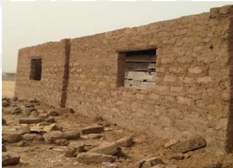
Figure 2.16: Rammed Earth Wall, (Ede et al., (2017).
