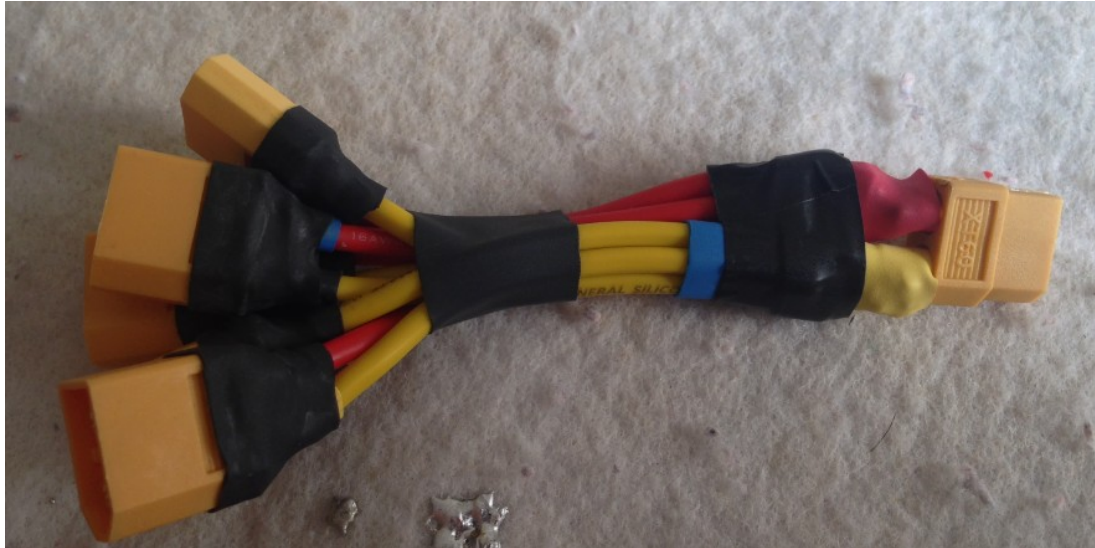
Figure 6.7: A bundle of power distribution cables are built to be used.
