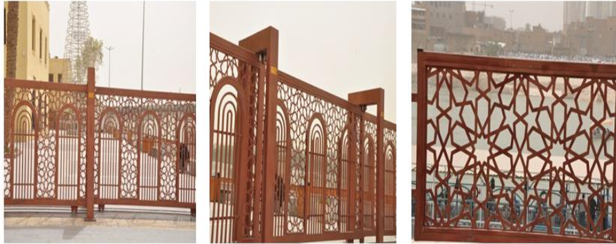
Figure 5-23 Iron fences from the Al-Qishla site in Baghdad. (Source: Researcher's photo).
