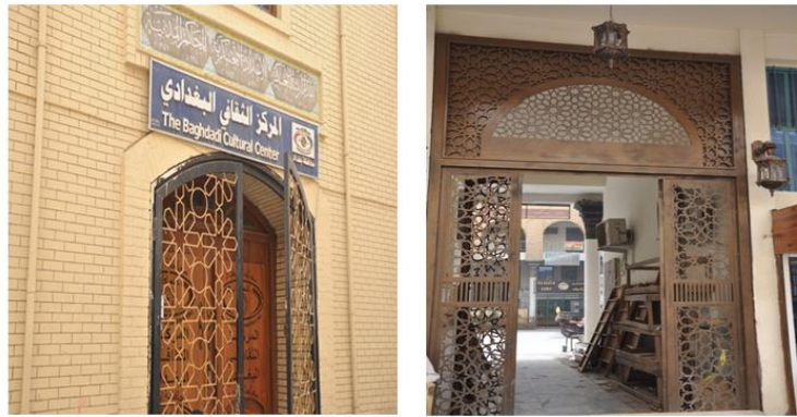
Figure 5-25 Iron doors designed according to Islamic motifs and shapes, Al-Baghdadi Cultural Centre. (Source: Researcher's photo).
