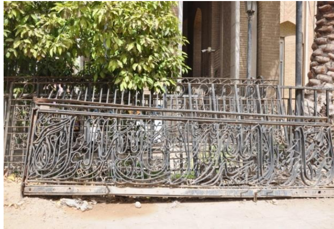
Figure 5-21 Iron balcony frame decorated with Holy Quranic verses, Al-Khulafa Mosque, Baghdad. (Source: Researcher's Photo).
