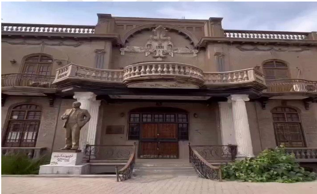
Figure 2.1. Front photo of Tawfiq Al-Suwaidi's house, architectural elegance and historical illumination, 2023 (The researcher).
