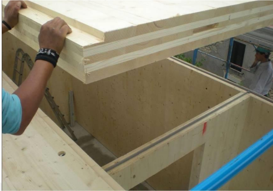
Şekil 4.5 Afet Konutu, Energy Box İtalya, L'Aquila (2009), Elektronik kaynak: https://www.treehugger.com/green-architecture/energy-box-earthquake-proof-passive-house-built-cross-laminated-timber.html
