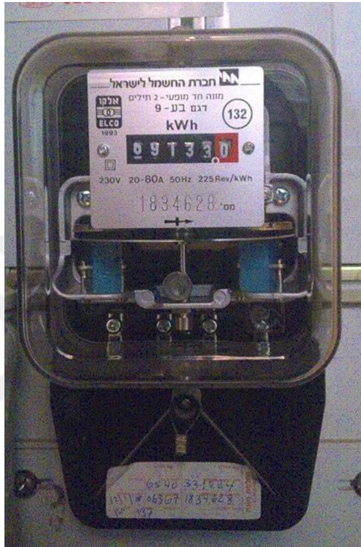
Figure 4.1: depicts a conventional electricity meter with one phase and two wires
