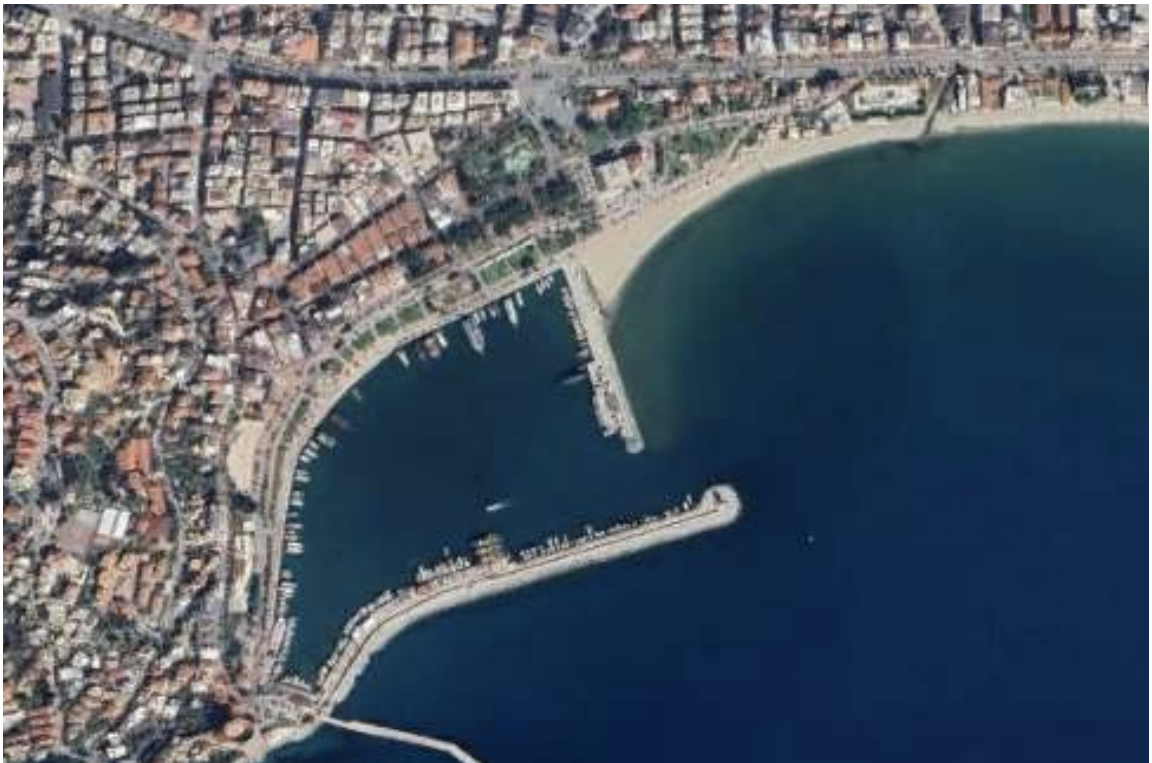
Figure 1.2. Concrete groin and sand accumulation.
