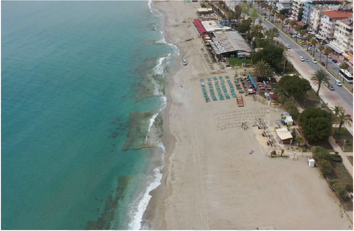
Figure 4.6. Image of exposed beach rocks from air.
