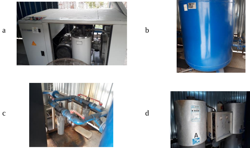
Figure 2.2 Cooling system a) compressor b) air tank c) filters d) dryer (Personal archive, 2019)
