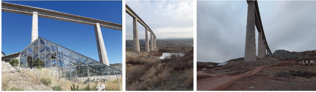
Figure 4.5 Views of high-speed train viaduct.
