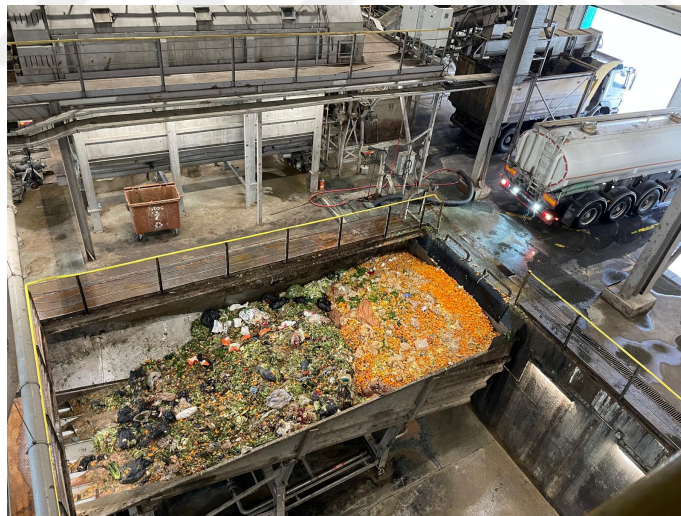
Figure 4.2. Waste collection site, Istanbul Metropolitan Municipality Kemberburgaz Biomethanization Plant.
