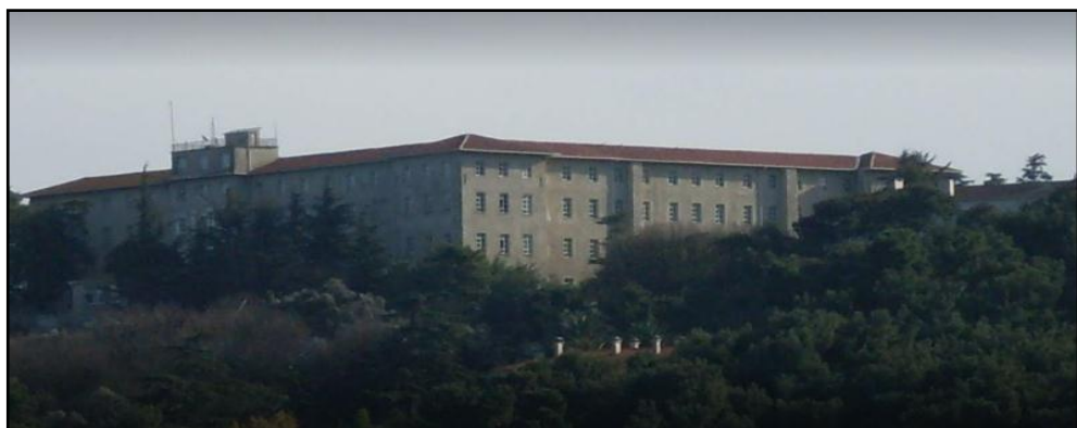
Figure 3.22. Recent building (The Elen Trade School) [18].
