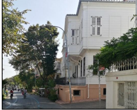
Figure 6.2. The electric pole on Refah Şehitleri Street [18].
