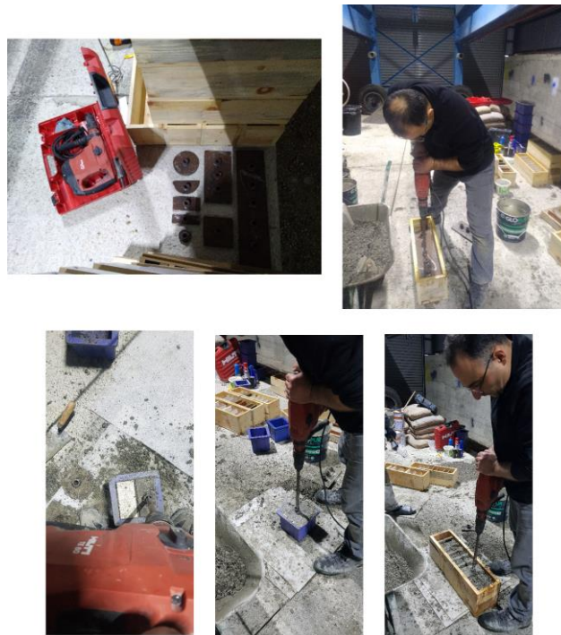
Figure 46. Apparatuses used in the sampling and compaction process of the fresh concrete
