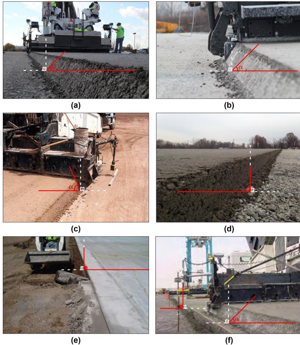
Figure 5. (a) Removal of a full-depth-trimmed unsupported edge of the first lane (creation of a right angle longitudinal cold joint), (b) Example of using an angled-paving-shoe as casting the second lift of two-layer RCCP (Harrington et al., 2010), (c) Example of using a different shoe type to create an acute-angled taper of the joint (Park et al., 2020), ( \alpha : the slope angle of the longitudinal joint)
