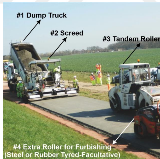
Figure 15. Consequent construction phases of an RCCP (adapted from Jofré (2019))
