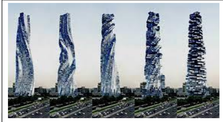
Figure 2.12 Rotating Tower in Dubai
