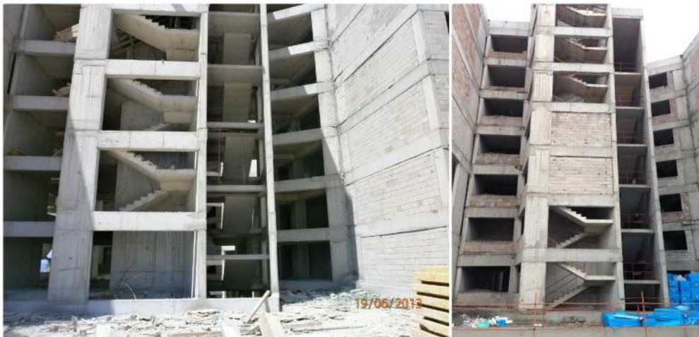
Figure 5.7. Guardrails in staircases (3)
