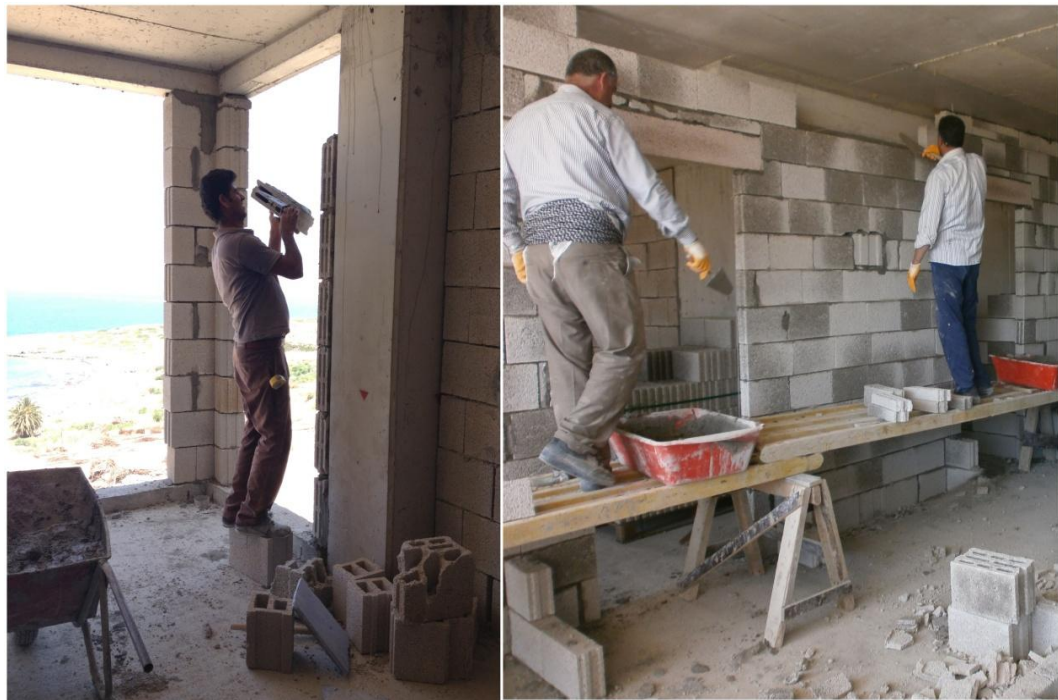
Figure 5.13. Work at height level
