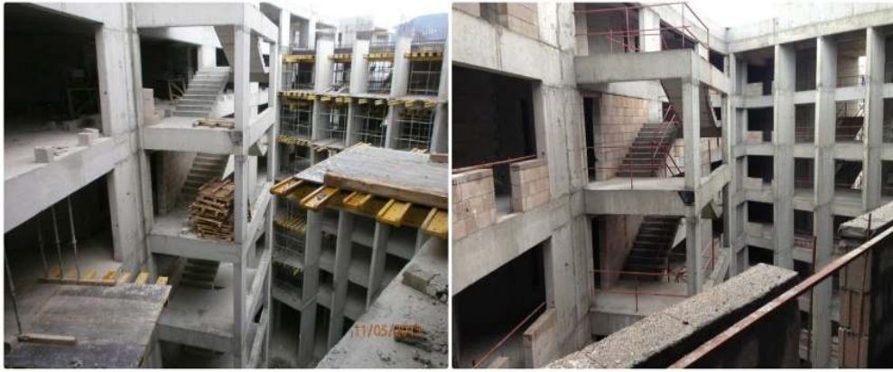
Figure 5.5 Guardrails in staircases (1)
