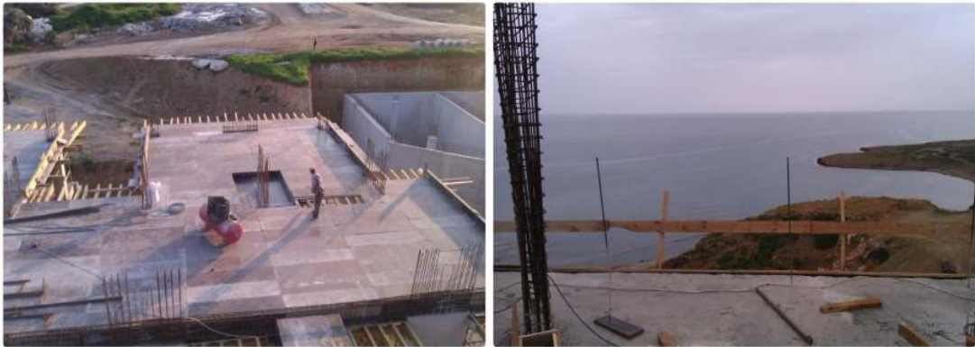
Figure 5.4. Guardrails in LPH project
