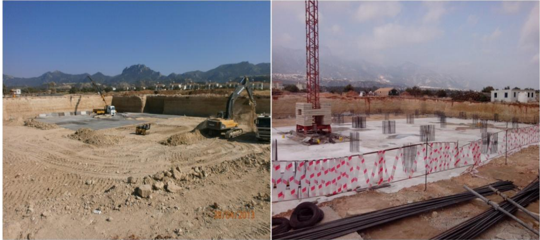
Figure 5.11. Warning line systems
