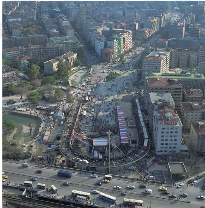
Figure 3.10. U-turn bridge constructed in 1997. Retrieved from:
