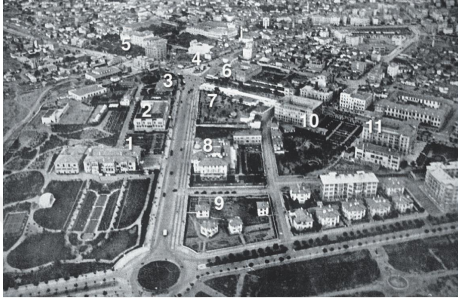
Figure 3.8. The aerial view of Ulu in 1930s. Number 7 shows Millet Bahçesi. (Kezer, 2015: 24)
