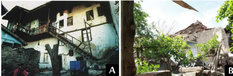
Figure 3. 9. The case study building CS04 in the early 1990s (Source: Şahin, 1995) (A) and its ruins in 2021 (B)
