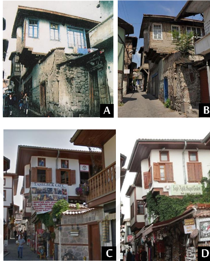
Figure 3. 3. The case study building CS01 in the early 1990s (Source: Şahin, 1995) (A); in 2011 from the street view of Yandex Maps (B); in 2018 taken from the street view of Google Earth Pro (C) and in 2021 (D)
