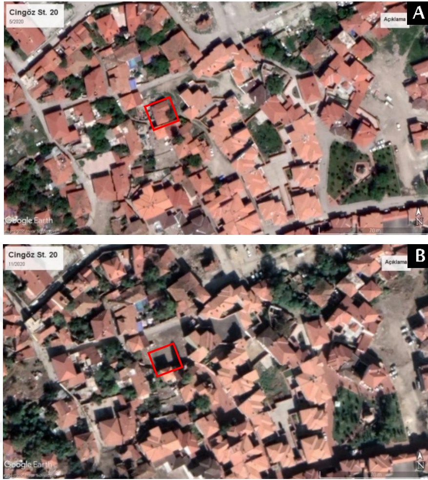
Figure 3. 7. The case study building CS03 in demolition process in 5/2020 (A), and 11/2020 (B), respectively, from Google Earth Pro
