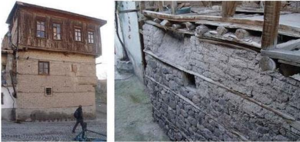
Figure 2. 2. Hımış technique (left) and timber lintels in the masonry (right) examples from GÜDÜL, Ankara. (Source: Şahin Güçhan, 2018)
