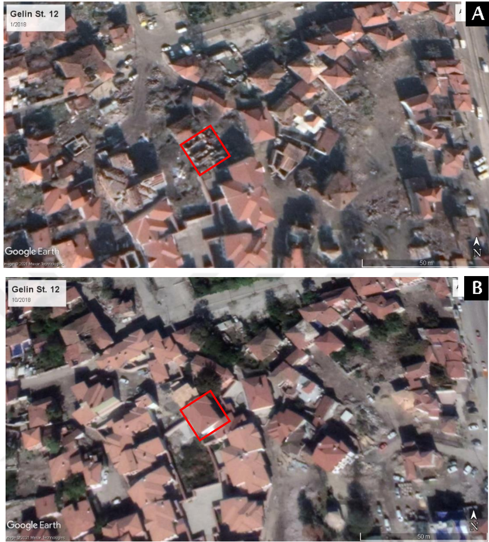
Figure 3. 12. The case study building CS07 in the reconstruction process in 1/2018 (A); in 10/2018 (B) from Google Earth Pro
