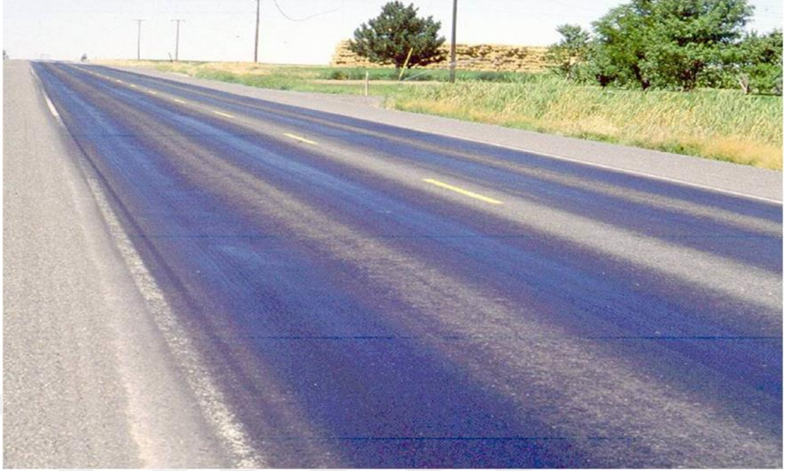
Şekil 2.20. Kusan Asphalt (Bleeding Asphalt)
