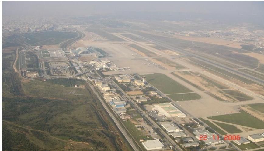
Figure 6.1 General view of Adnan Menderes Airport
