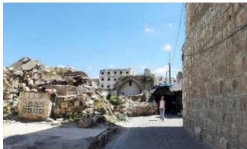
Demolished buildings because of bombing
