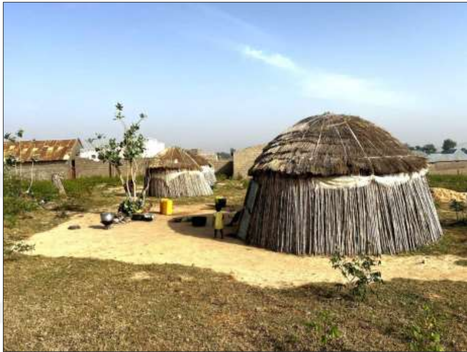
Figure 4.8: Hut Housing in Some Parts of Zamfara State (Author, 2024)..
