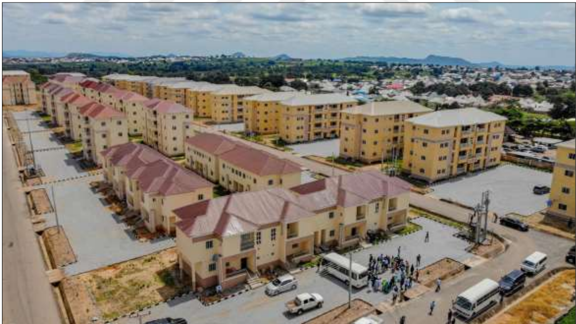
Figure 3.10: Mass Housing Unit in Abuja (TechCabal).
