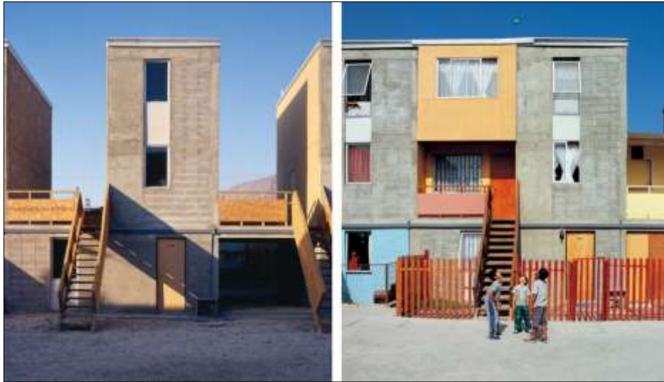
Figure 2.19: Quinta Monroy Housing Project (Carrasco & O'Brien, 2021).
