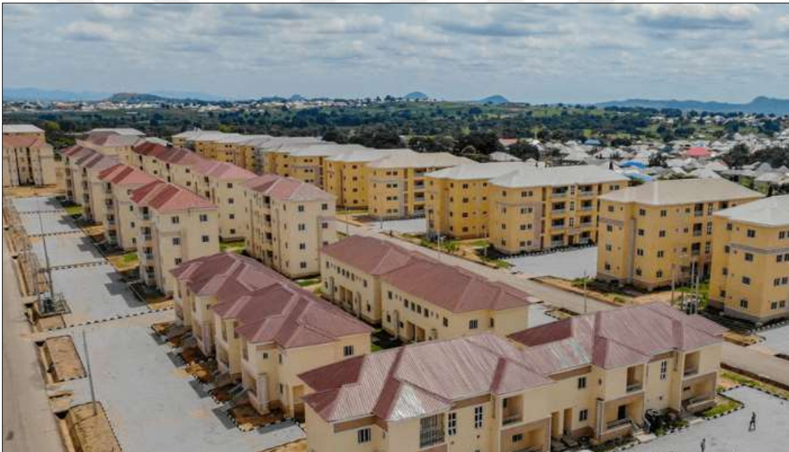
Figure 3.7: Social Housing by Ministry of Work in Zuba (Niarametrics).
