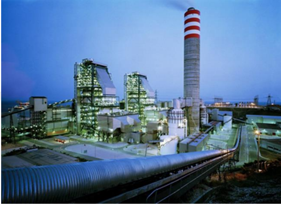
Figure 3.1. A view of the steam power plant (ISKEN 2018)
