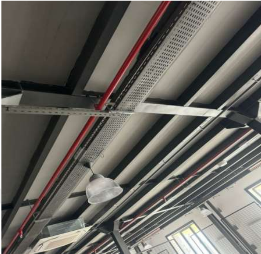
Figure 3.21 The roof of Studio Room 1 of Samsun University.
