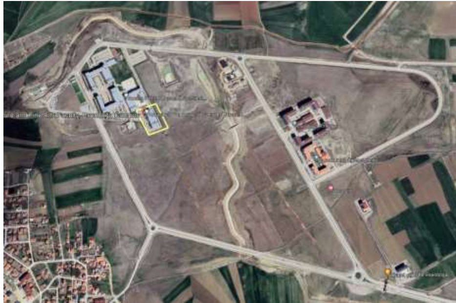
Figure 3.25 AYBU Architecture Department site topographic location
