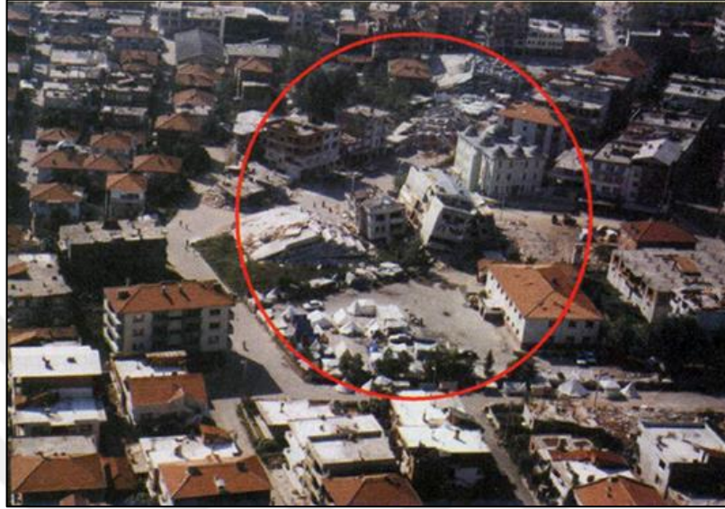
Figure 2.2 Liquefaction damage on buildings (Kocaeli Earthquake, Adapazarı 1999, Photograph by Ömer Aydan)
