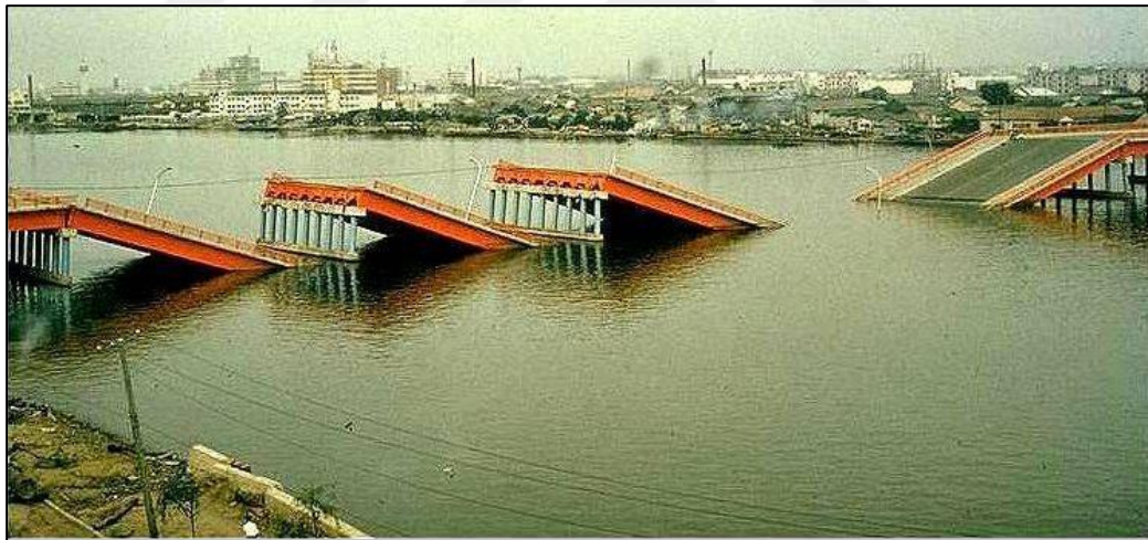
Figure 2.4 1964 Niigata Earthquake; Showa Bridge (Kramer and Elgamal, 2001)
