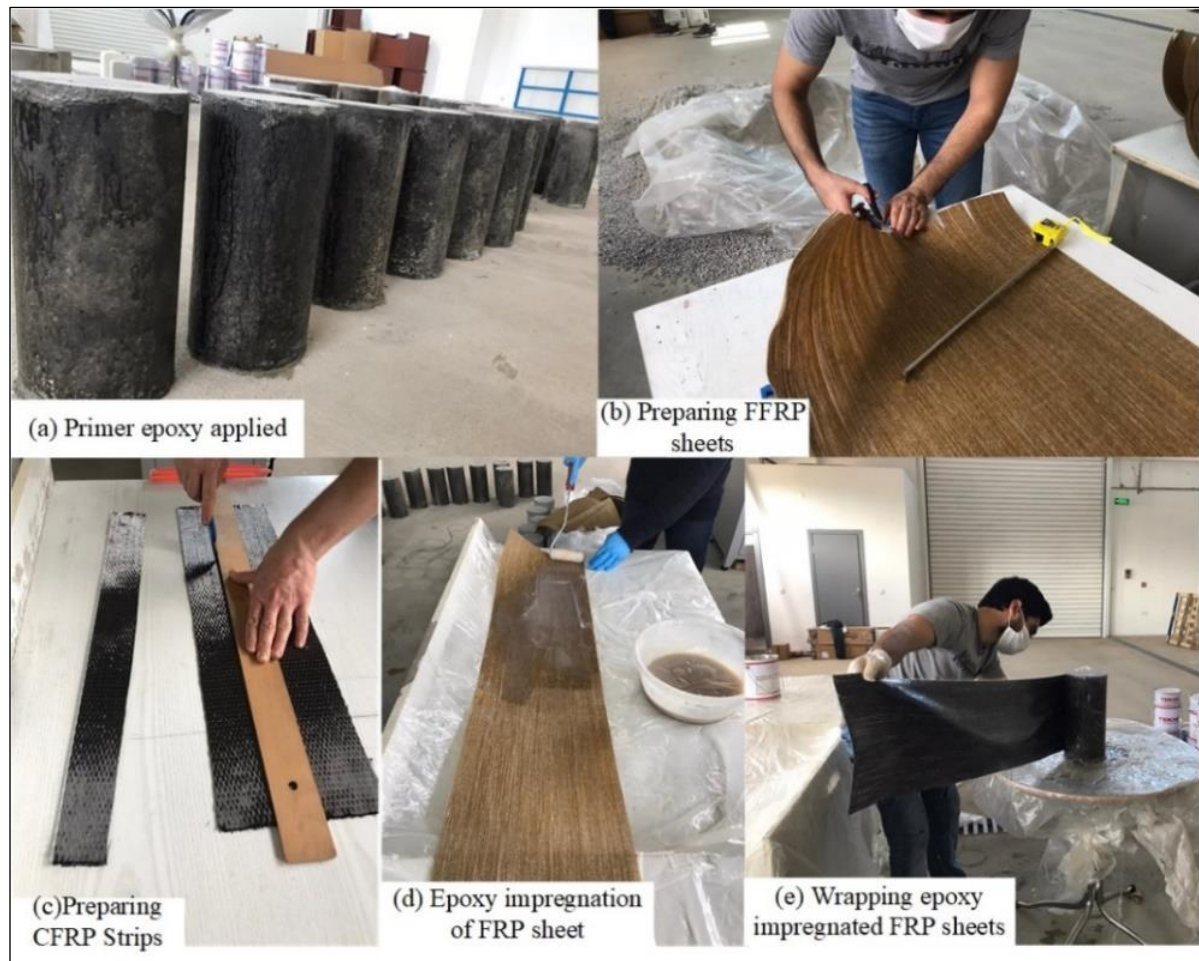
Picture 3.4 FRP confinement procedure
