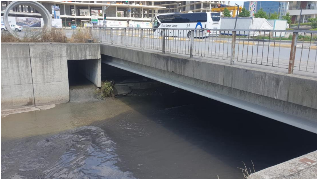
Figure 3-20 View near the bridge at the station 10050 meters
