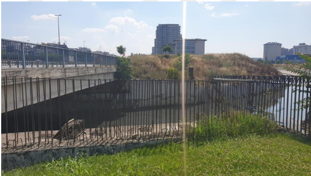
Figure 3-17 View near the bridge at the station 3250 meters
