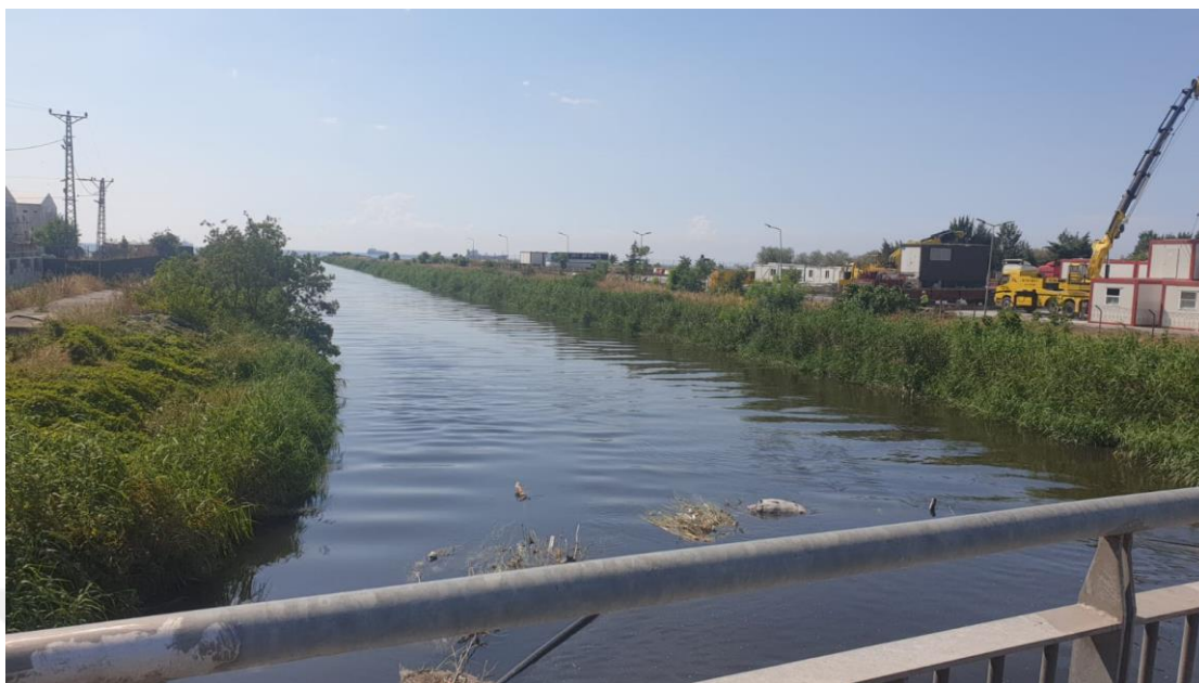
Figure 3-14 View over Bridge at the station 22 meters
