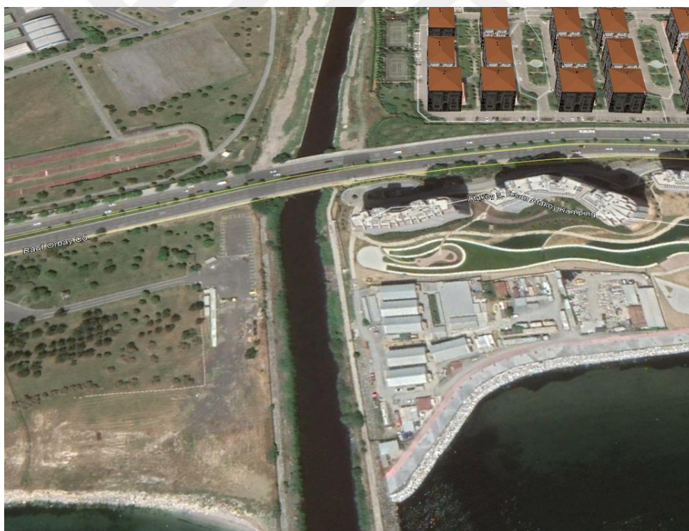
Figure 3-15 Google Satellite View at the bridge station 22 meters
