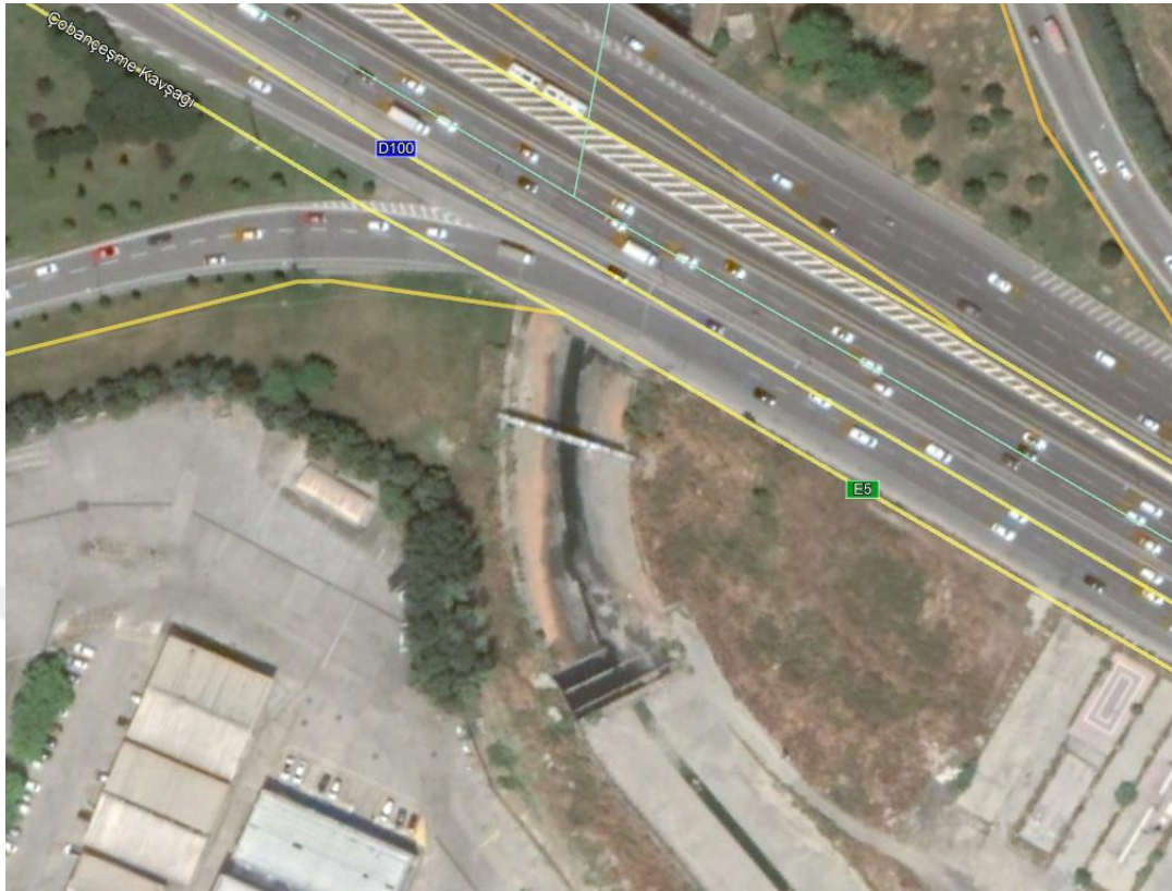
Figure 3-18 Google Satellite View at the bridge station 3250 meters
