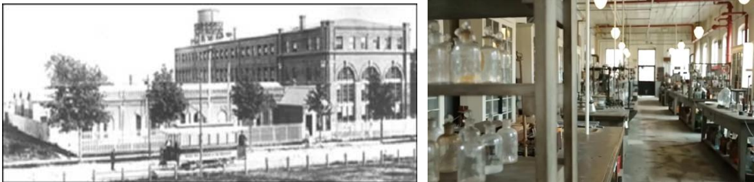
Görsel 4.9. Edison West Orange Laboratuvarı, New Jersey (Millard ve Carlson, 1987)
