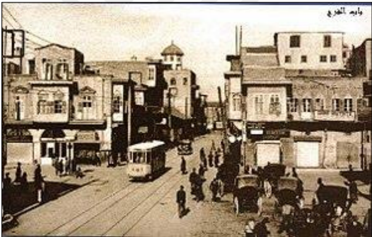
Figure 3.5: Tram Line, Put Into Operation in 1929 (Dig-doc.org, 2006).
