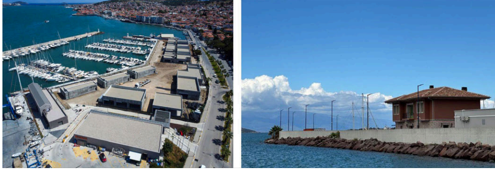
Figure 3.14 Marina started to be constructed along the coastline. Source: ATP.
