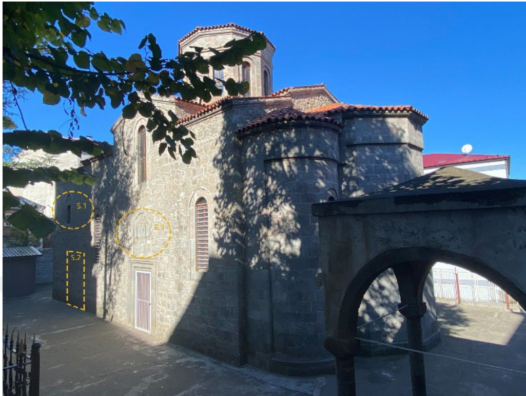
Figure 4.4. South facade of the church St.John Exoteichos (Gönülnur Demet, 2022)
