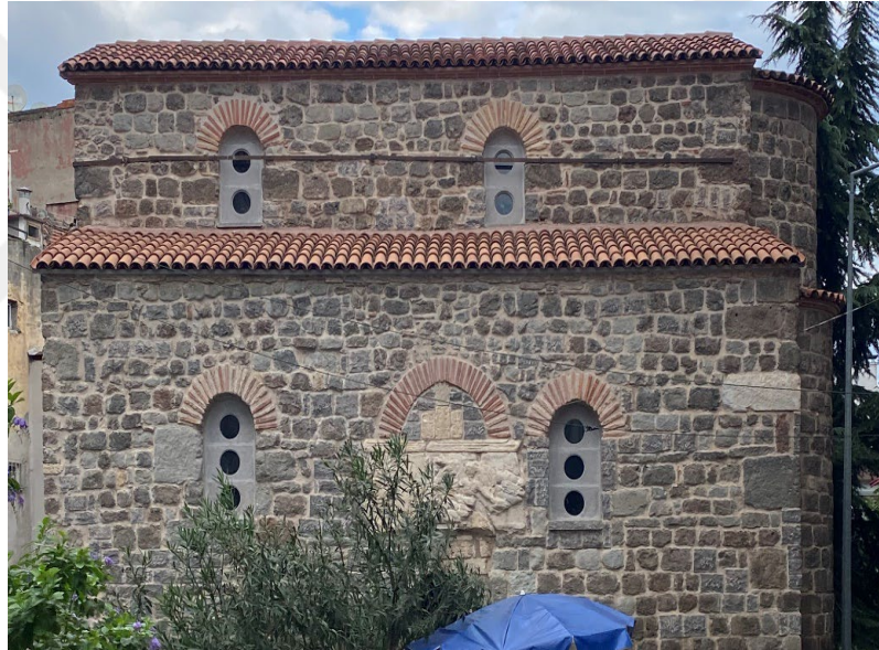
Figure 2.9. The south façade of Church of St. Anne in 2022 (Note: Gonulnur Demet, The south façade of Church of St. Anne in 2022)
