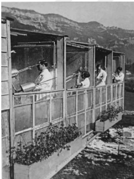
Figure 170. Jean Saidman, revolving sanatorium, Aix-les-Bains, France, 1930
