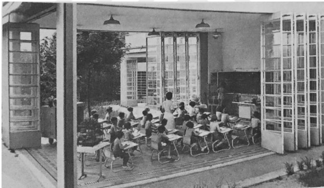
Figure 184. Classroom with retractable walls
