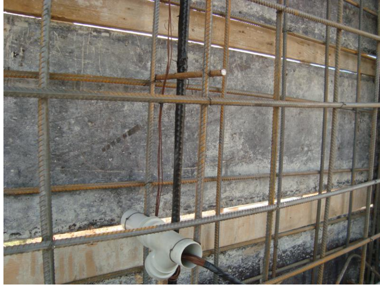
Figure 3.22 Fixing of thermocouple wires in their positions
