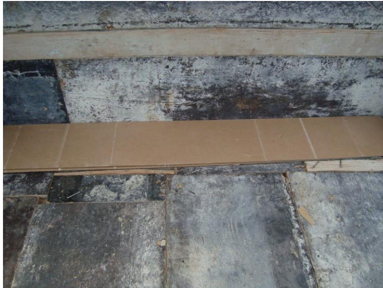
Figure 3.4 Two layers of plywood on the top of concrete beams to thermally isolate the beams from the box-girder bottom slab
