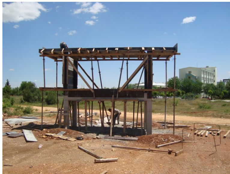
Figure 3.3 Formwork of the box-girder segment on the supporting frame
