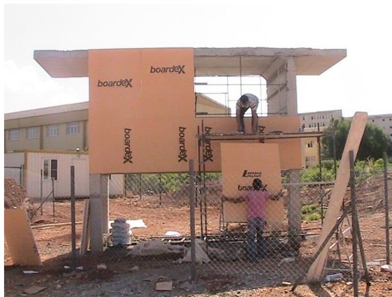
Figure 3.5 Installation of the isolation boards
