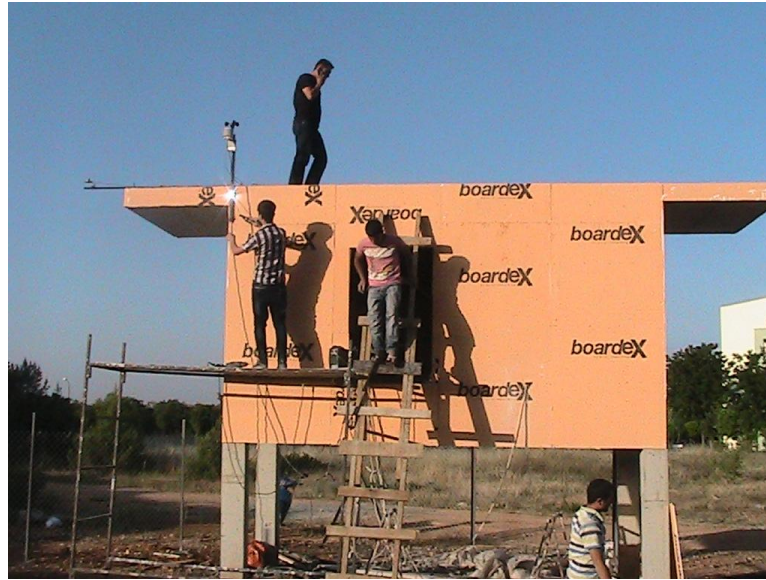
Figure 3.25 Installation of the environmental sensors in their permanent location
