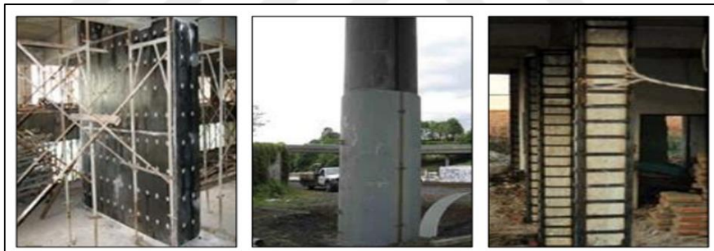
Figure 2.7 Steel angles and plates fixed around column [22]
