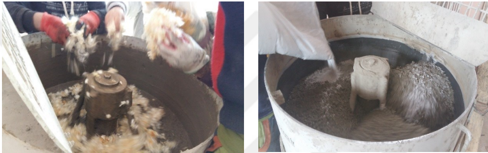
Figure 3.7 Mixing of materials
