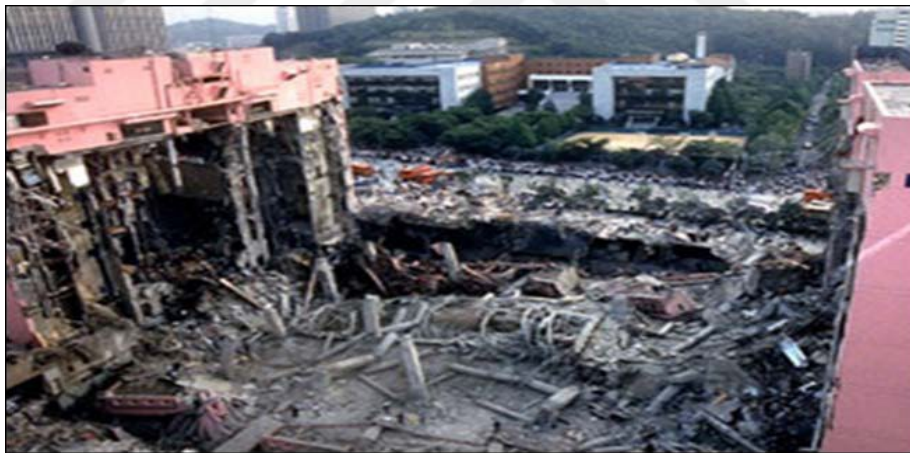
Figure. 1.4 Post-collapse photograph of the Sampoong Department Store
