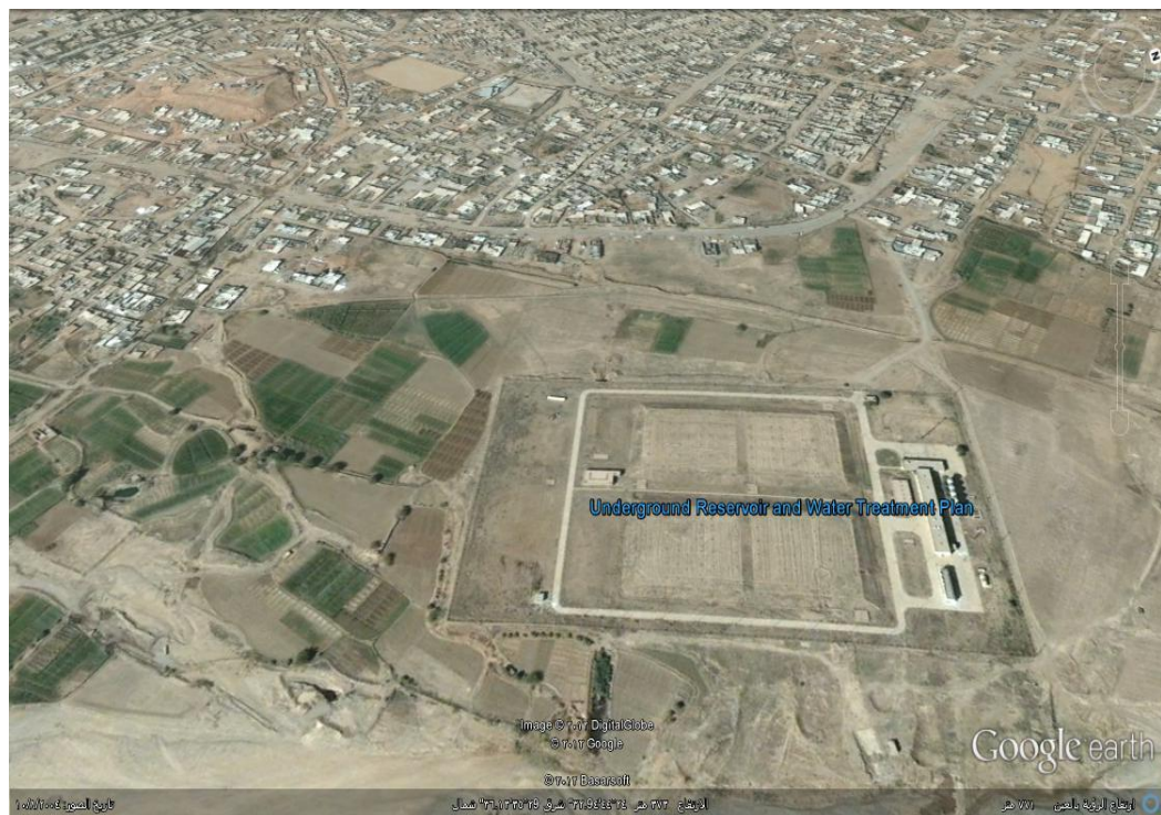
Figure 1.5 An underground Reservoir
