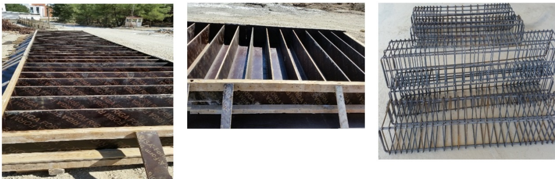
Figure 4.6. Producing of test specimens.
