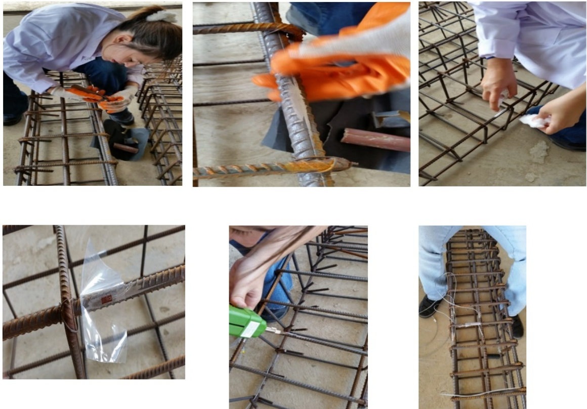
Figure 4.7. Installation of strain gages.
