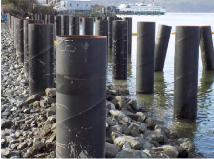
Figure 2.19 Steel piles at shore (Geo-Minds, 2023)
