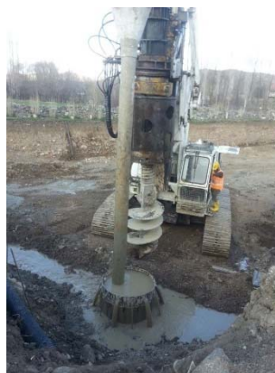
Figure 2.22 Piling in cohesionless ground (Geo-Minds, 2023)
