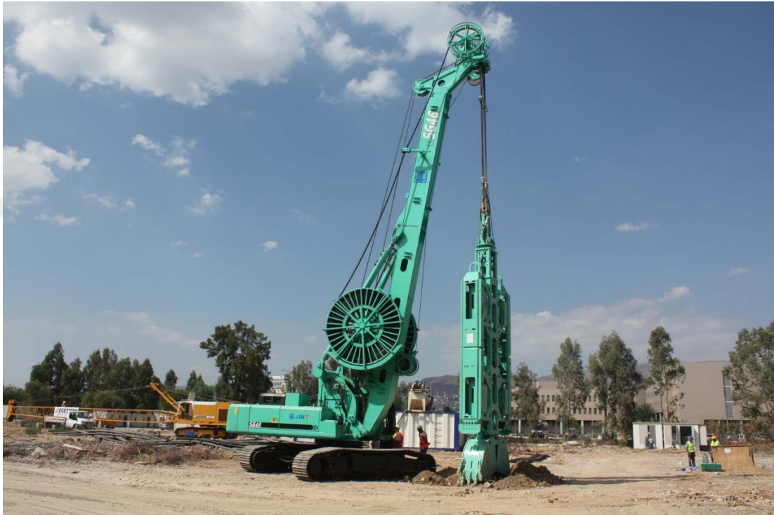
Figure 2.21 Barrette pile machine (Ege Zemin, 2023)
