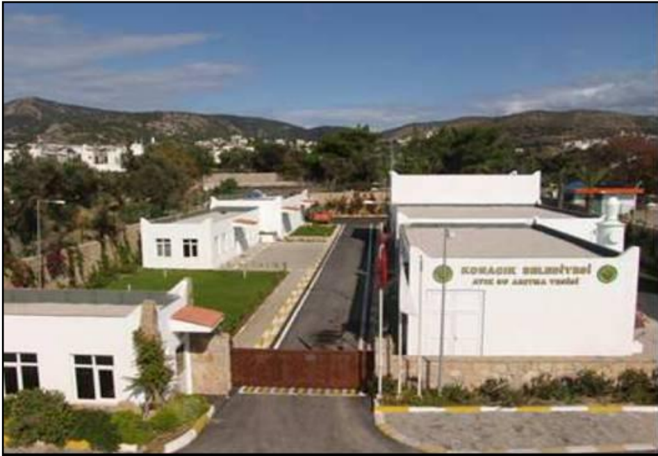
Figure 3.1 General view of Konacık wastewater treatment plant
