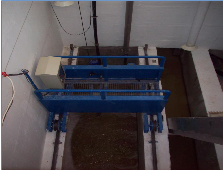
Figure 3.5 Grid collector mobile bridge
