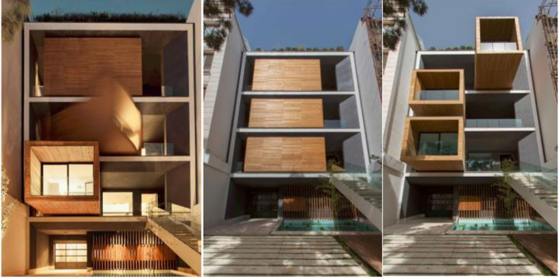
Görsel 3.35 Sharifi-ha House, 2014 (http-44)
