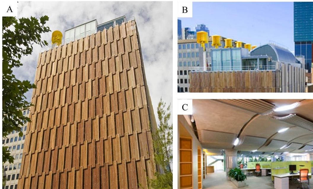
Figure 33: (A) Front Façade of Melbourne CH2 Building. (B) Using a Microturbine and Solar Panels, CH2 Produces Electricity, Hot Water, and Cooling on its own. (C) CH2 is able to Sustain Thermal Comfort in both the Summer and the Winter thanks to Energy-Efficient Heating and Cooling Technologies. Source: (City of Melbourne, 2006)
