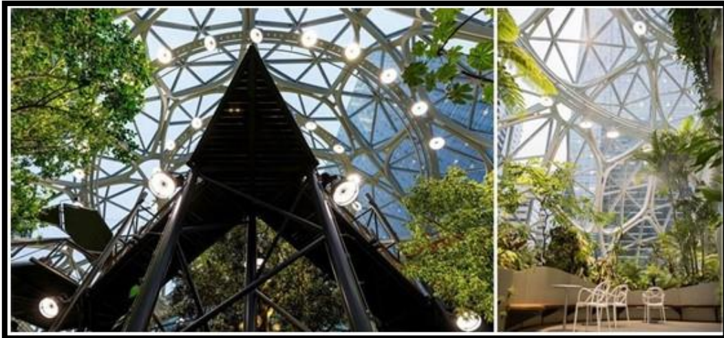
Figure 4.18: Photos Of The Lighting System In Amazon Spheres [97].
