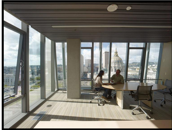
Figure 2.5: An Opening Window In The Meeting Room For Ventilation [19].
