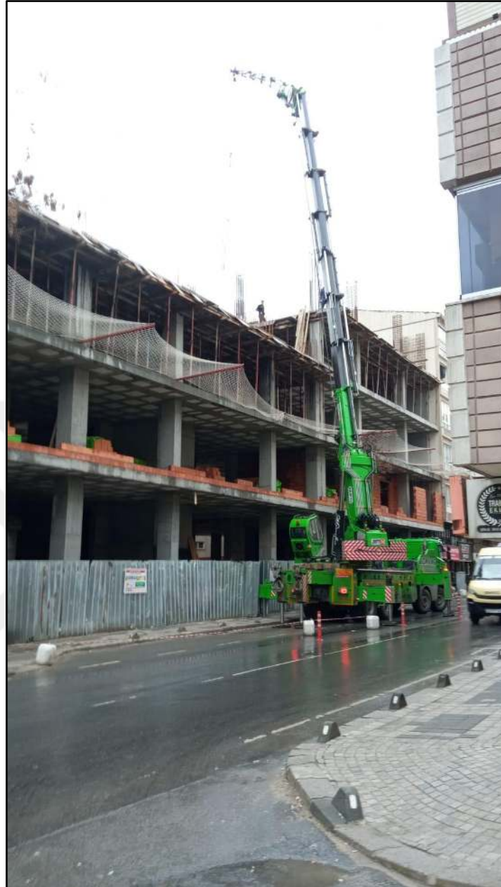
Figure 1.2: A Mobile Crane Hoisting a Load Much Below Its Capacity.
