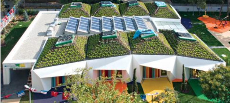
Figure 5.12 Green roof on Bahriye Üçok Kindergarten
