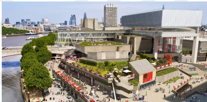
Figure 4.31 Green roof on Southbank Centre ( https://www.archdaily.com/tag/southbank-centre ) [Accessed 30.04.2021]
