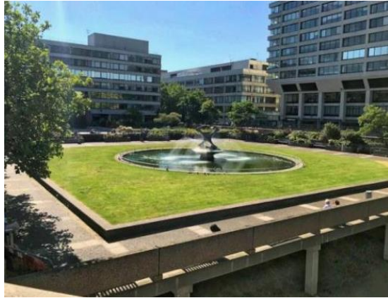
Figure 4.29 Green roof on St Thomas's Hospital
