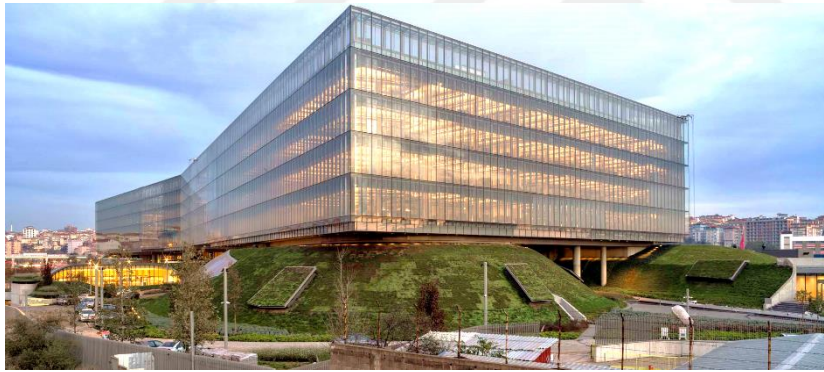
Figure 3.53 Green roof on Garanti Bank Technology Campus
