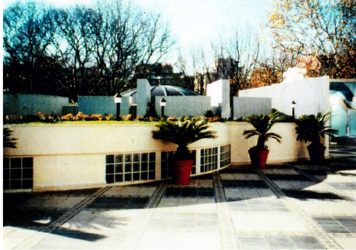
Figure 5.3 Green roof on Ceylan International Hotel (Köylü, 1997)
