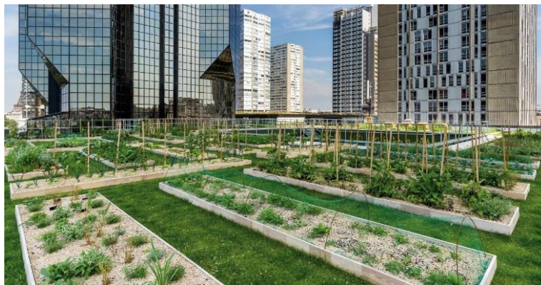
Figure 3.40 Planting beds on green roof ( https://zinco-greenroof.com/press-release/le-cordon-bleu-paris ) [Accessed: 10.12.2020]
