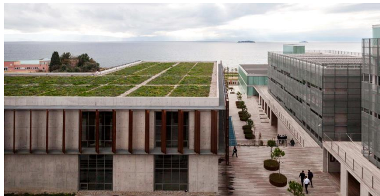
Figure 3.52 Green roof on Piri Reis University
