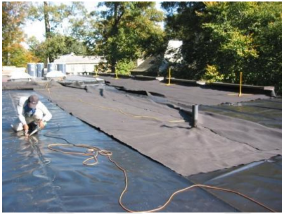
Figure 3.24 Root barrier
