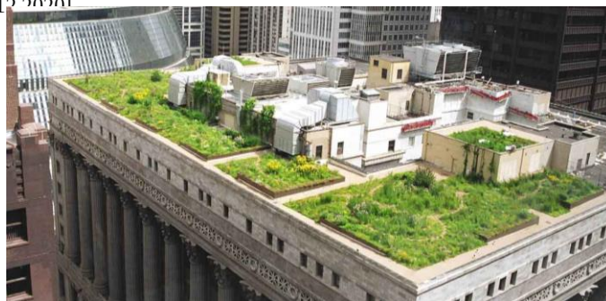
Figure 3.43 Green roof in Chicago City Hall
