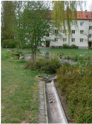
Figure 2.4 Stormwater canal at the Eco City Augustenborg
