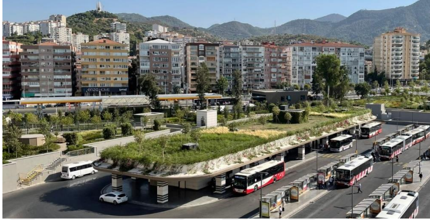
Figure 5.18 Green Roof on Üçkuyular Terminal
