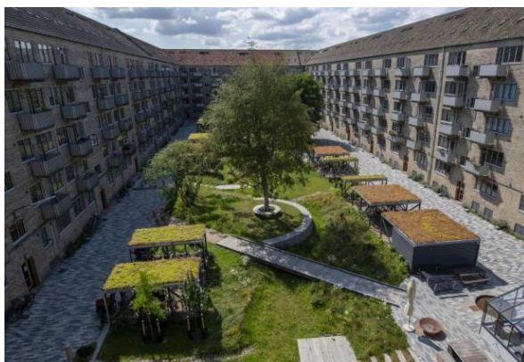
Figure 4.25 Green Roof on open-sided huts ( https://www.kk.dk/nyheder/nu-indvies-fremtidens-gaardhave-i-askoegade ) [Accessed: 28.12.2020]
