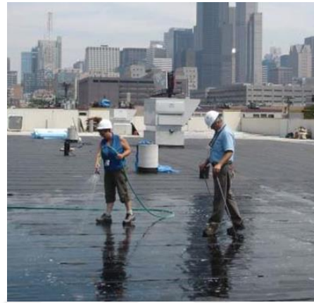
Figure 3.25 Waterproof membrane
