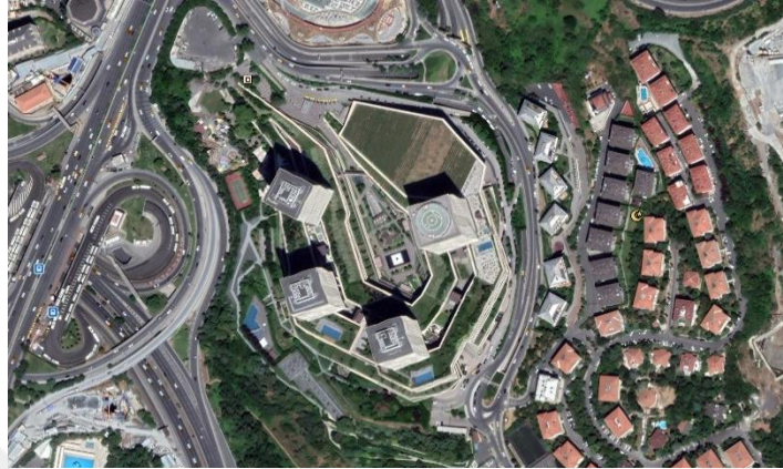
Figure 5.8 Aerial view of Zorlu Center (Google Earth, 2020)
