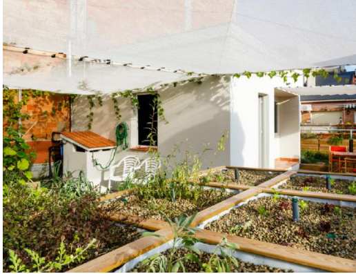
Figure 4.2 Green roof in the street of Balcells
