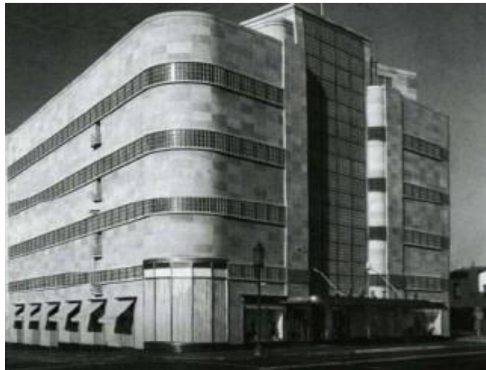
Şekil 28- Clements, Coulter’s Department Store, Los Angeles (Mülayim, 2017).
