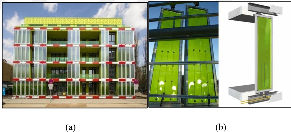
Figure 2.13. (a) BIQ House, (b) microalgae on glass panels [30].
