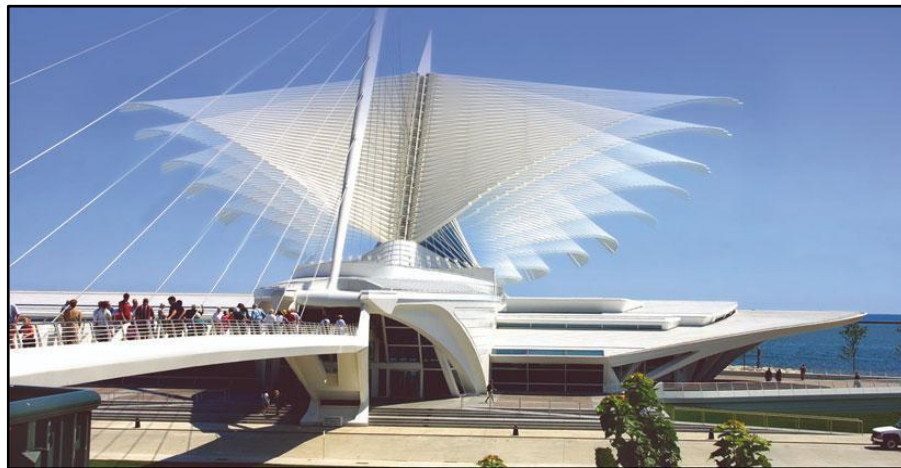
Figure 2.32. Milwaukee Art Museum dynamic roof system [66].
