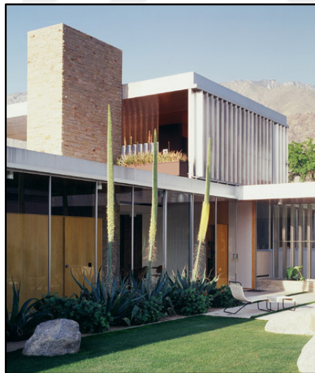
Figure 3.20. The hand-operated facade of the Kaufman House [115].
