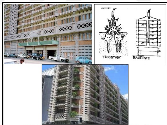
Figure 4.4. Relation between Eastgate building and termite tower [45].
