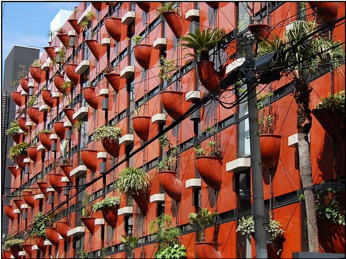
Figure 3.2. Organic Building, Osaka, Gaetano Pesce, 1993 [34].
